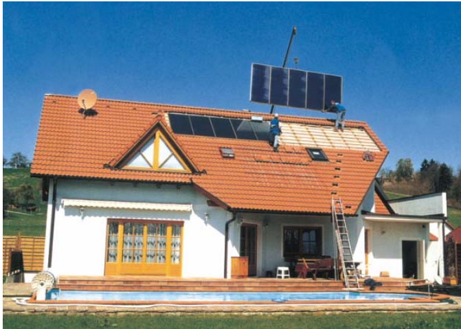
Fig. 4: Mounting collector modules with a crane
