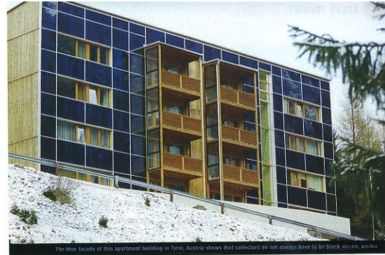
The new facade of this apartment building in Tyrol, Austria shows that collectors do not always have to be black either. AUSTRIA
